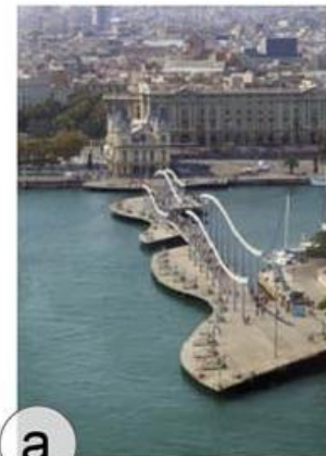
a Barcelona Bridge
